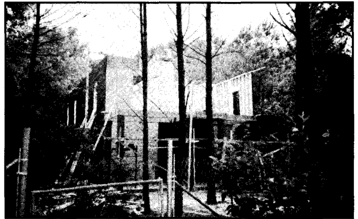
Construction on the new Research and Education Building is well underway.
