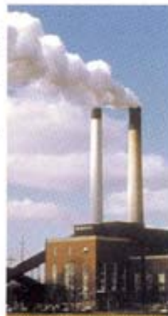
Coal fired power plants are the primary source for atmospheric mercury worldwide
