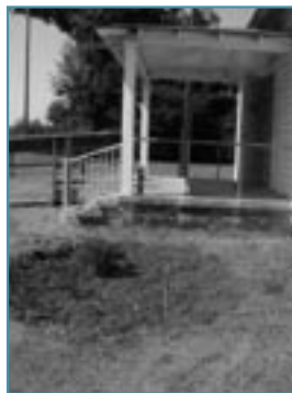
Newly installed rain garden designed to capture rainfall runoff for the Sonora Community Hall roof
