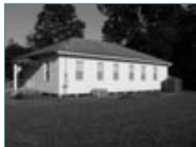
Rainfall collected by the cistern at rear of the Sonora Community Hall will be used to irrigate the adjacent raised garden
